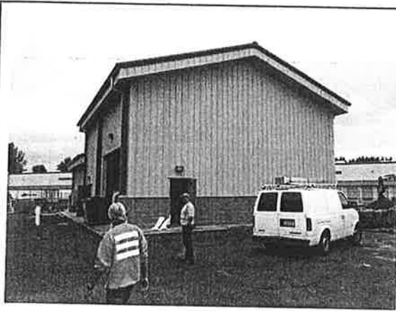
Central Well Building
