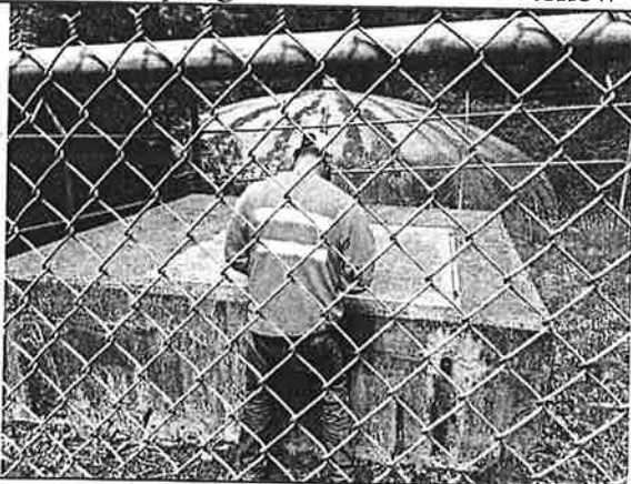
Sumner Springs Weir Vault
