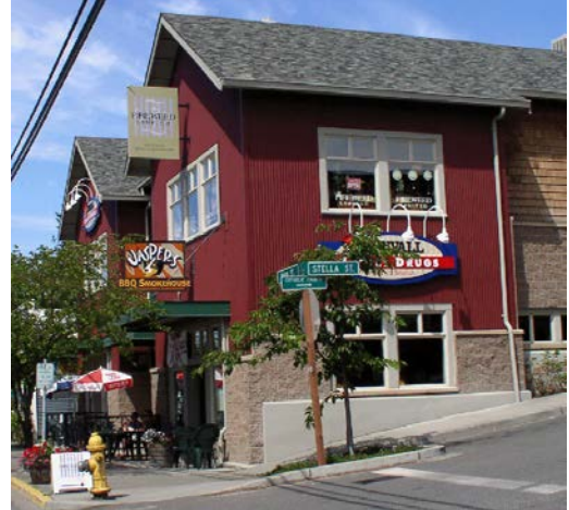
Figure 2-34. This building features metal siding with visible corner trim and concrete block closer to the ground level.
