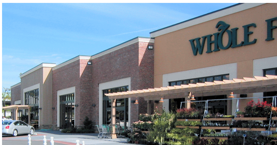
Figure 2-26. This building uses a combination of material changes, modulation, a distinctive window pattern, and a trellis to reduce its perceived scale and add visual interest.
