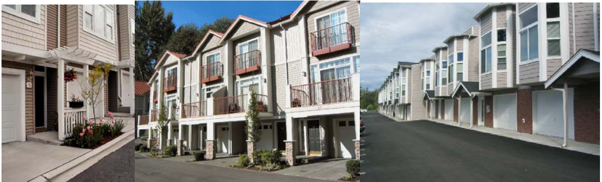
Figure 3-7. Good and bad examples of garage/entry configurations. The left example features a landscaped area and a trellis to highlight the entry. In the middle image, the balconies and landscaped areas deemphasize the garage. In the right image, the lack of landscaping is a glaring omission.
