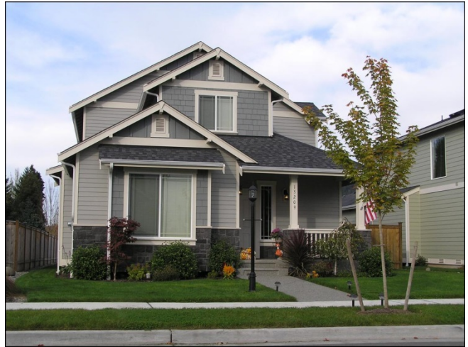
Figure 4-13. This homes includes stonework detailing, decorative roofline elements (multiple gables), decorative siding (shingles), and roof brackets.
