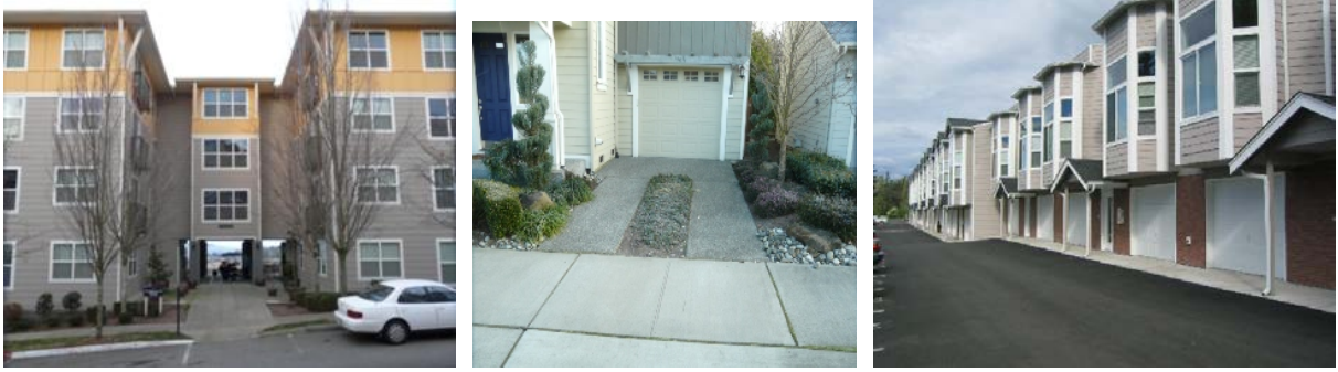
Figure 3-14. Good and bad examples of garage/entry configurations. The left example features a courtyard area and benches to highlight the entry. In the middle image, the increased setback and landscaped areas deemphasize the garage. In the right image, the lack of landscaping is a glaring omission.
