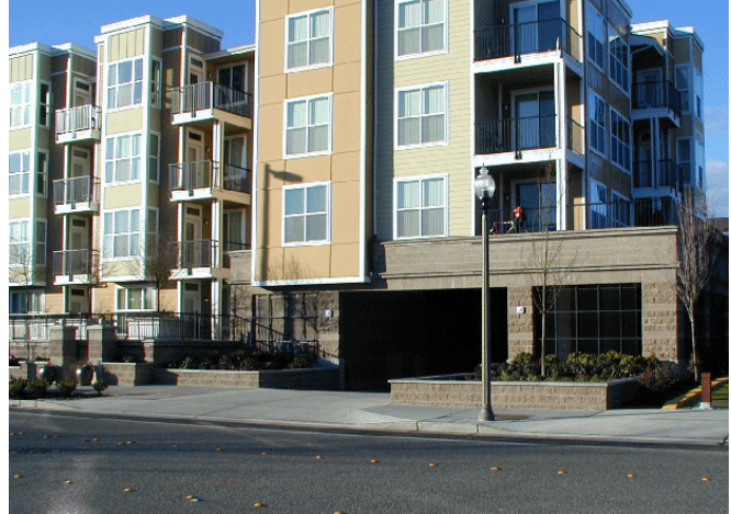
Figure 3-20. This parking garage is clearly visible, but doesn't negatively impact the character of the building.
