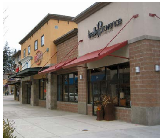
Figure 2-33. An example of concrete block effectively used with EIFS (see Guideline 2.4.6 below) and metal awnings.
