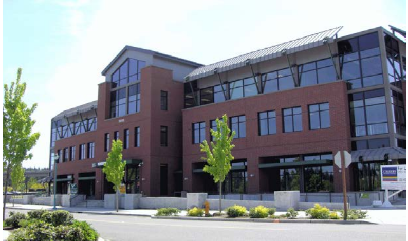
Figure 2-28. Acceptable alternative design treatment for a building wider than 120 feet. Note the entry's clear vertical and horizontal modulation elements.
