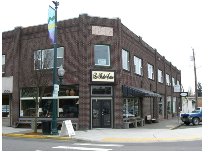
Figure 1-19. Brick is the preferred exterior material for the Historic District buildings.
