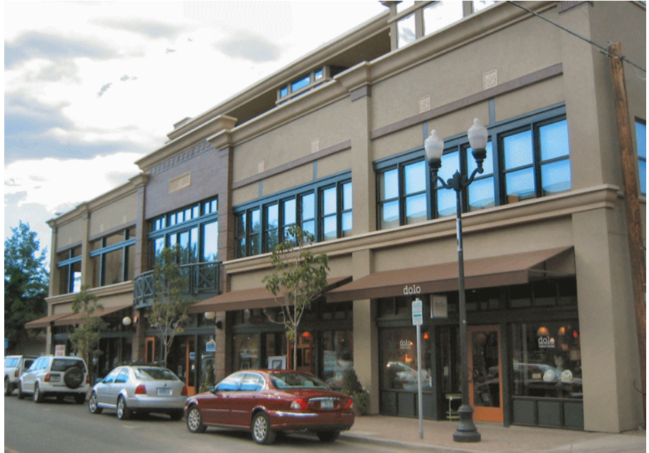
Figure 1-14. This building uses a clear change in building materials and other articulation techniques to reduce the perceived scale of the building and add visual interest.
