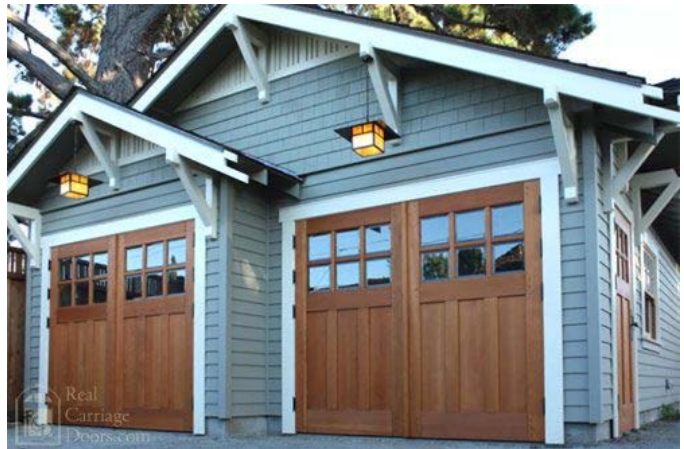
Figure 4-16. Good example of a garage design, where facing the street. Note the garage door detailing.
