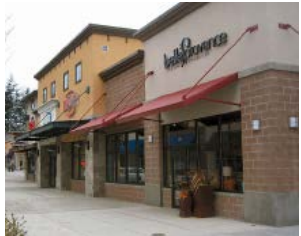
Figure 1-131. An example of concrete block used in conjunction with other materials.
