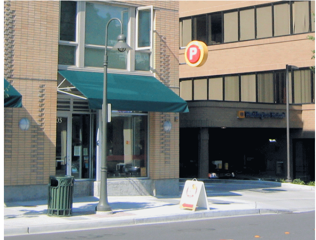
Figure 2-10. The parking garage for this mixed-use building is tucked behind the facade of the building and advertised with a simple sign and driveway.
