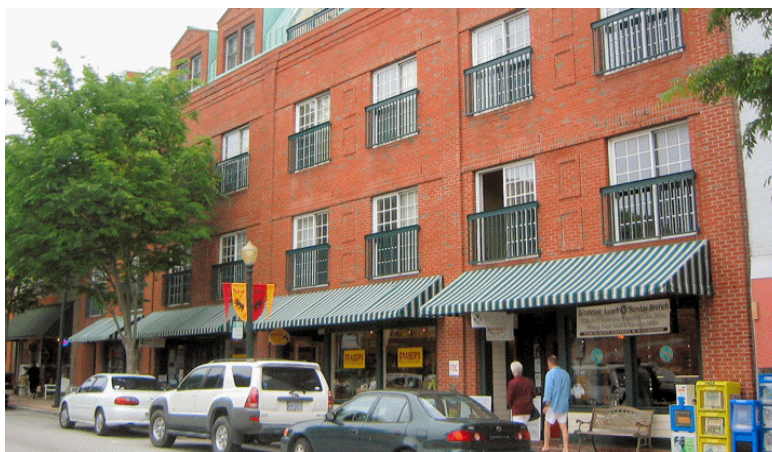
Figure 2-17. The multiple awning configuration on this building helps to articulate the facade and add visual interest to the building.
