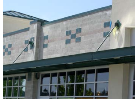
Figure 1-120. When concrete block is used on a facade, the design should utilize a combination of textured surfaces and color.
