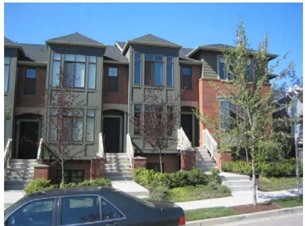
Figure 3-11. Another acceptable townhouse building. Note the landscaped front yards and individual walkways and entries. The internal units each have distinct, but identical windows and roof forms. The outside unit is differentiated through the use of building materials, window design, unit size, and facade detailing.
