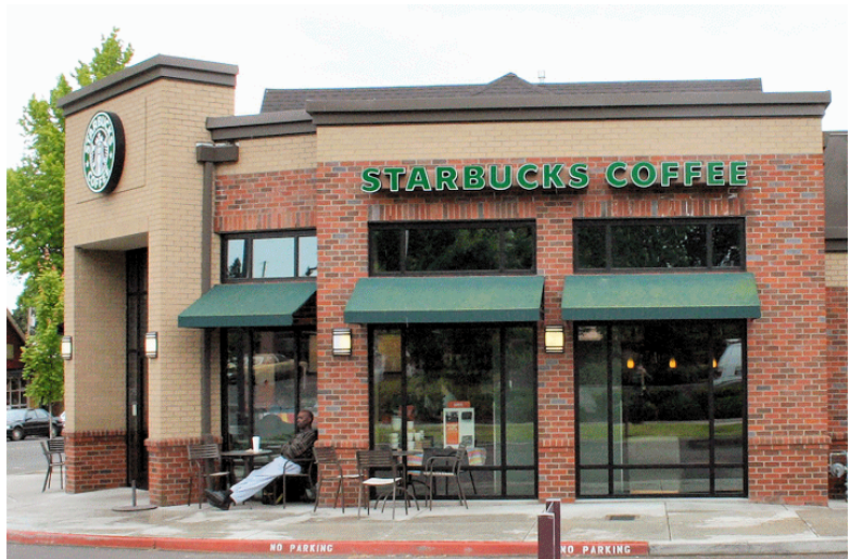
Figure 2-32. This building would meet the details guideline by using a decorative entry element, building materials, and lighting.
