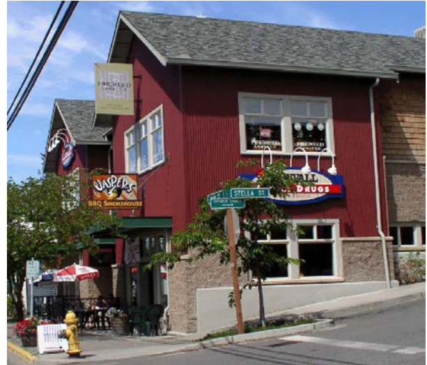
Figure 1-22. This building features metal siding with visible corner trim and concrete block closer to the ground level.
