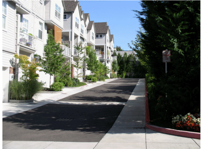
Figure 3-8. A well-landscaped alley
