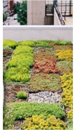
Figures 1-29. Green roof example.
