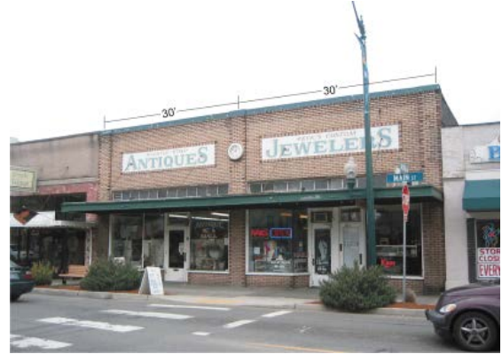
Figure 2-24. For commercial buildings built up to the sidewalk, provide facade articulation features at no more than 30-foot intervals.
