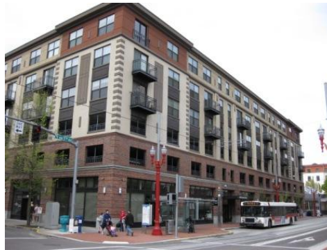
Figure 3-41. Illustration where CMU is used as a design element rather than a bland façade treatment.
