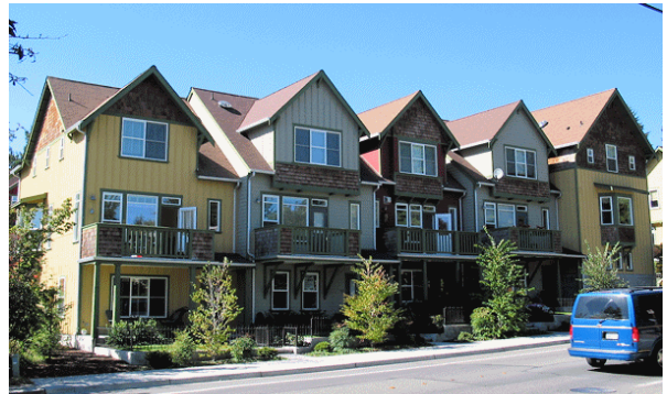
Figure 3-10. An acceptable townhouse example for Sumner. Note the varying façade treatments and colors, balconies, semi-private outdoor spaces, and street access.
