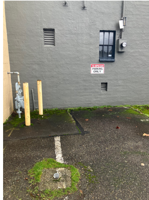
Underground tank to be decommissioned and removed
