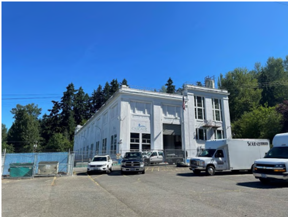
Photo 8 View of the northwest-adjointing White River Hydroelectric Power Plant (2111 East Valley Highway East), located northwest of Parcel B, from the northwest-adjointing property facing north.
