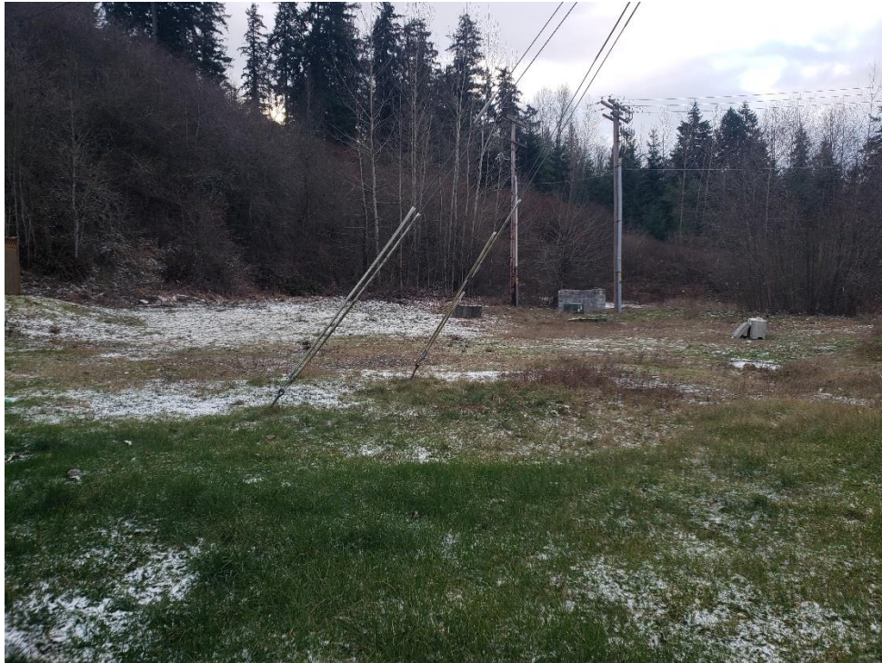
Photo 9 View of the southwestern portion of Parcel B, facing south from Parcel B.
