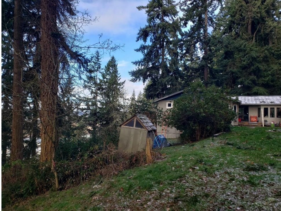
Photo 15 View of the north-adjacent properties to Parcel C (1705 & 1721 E Valley Highway E), facing north from Parcel C.
