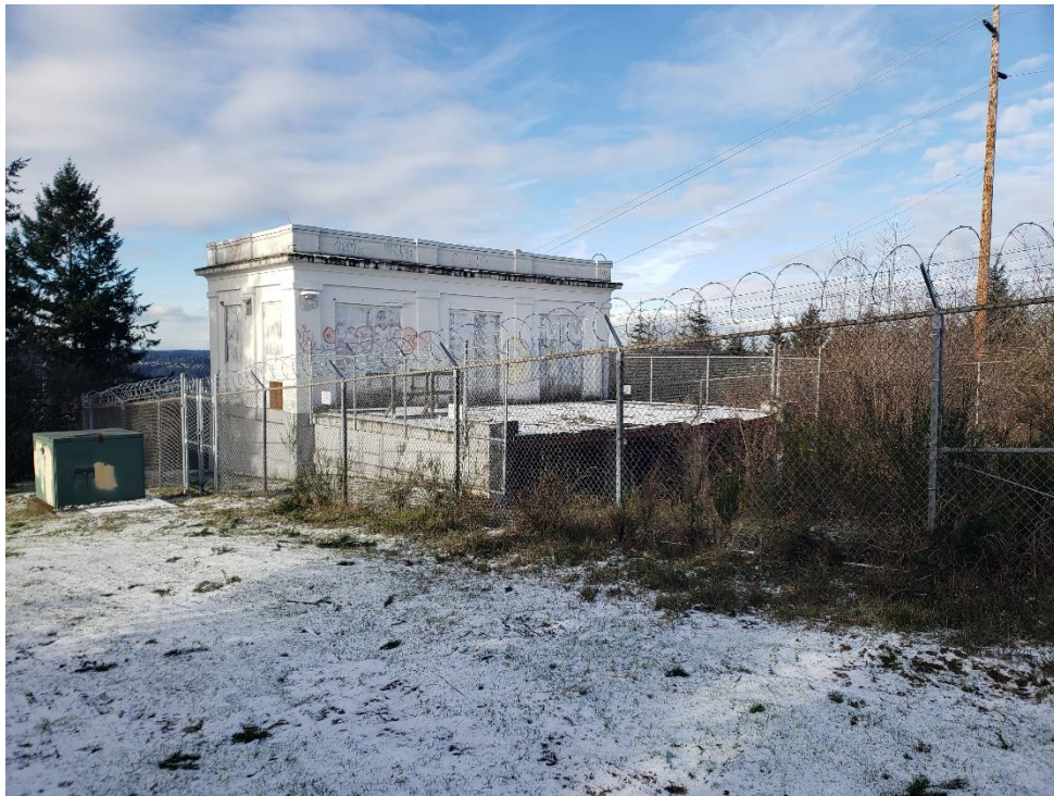
Photo 12 Typical view of a Cascade Water Alliance equipment building on Parcel B.
