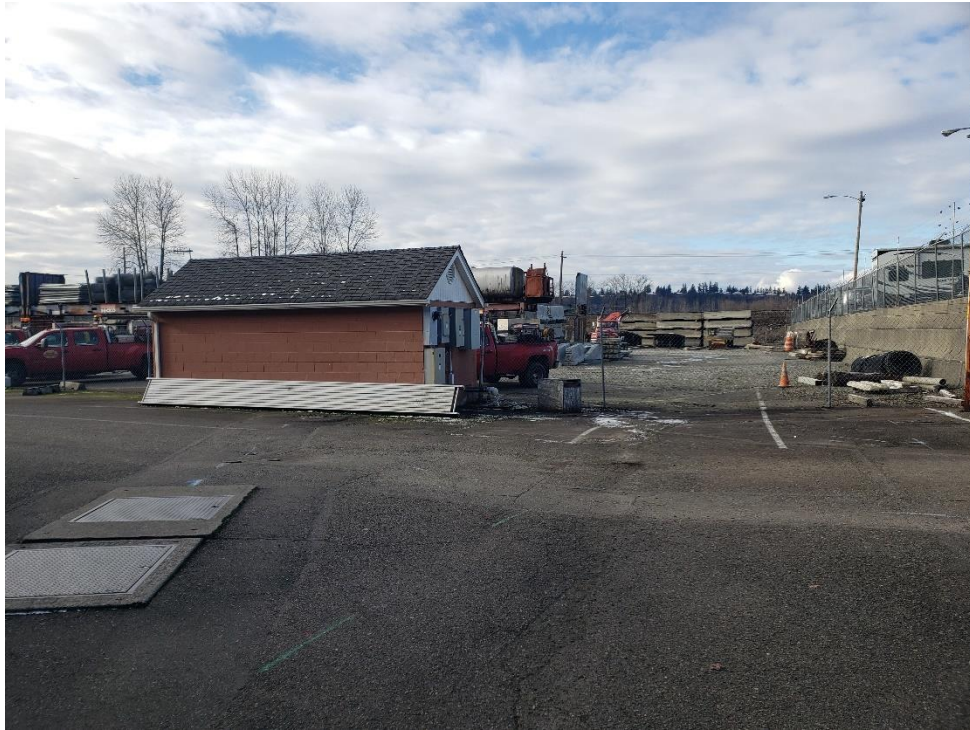
Photo 5 Typical view of the City of Sumner well pump house on Parcel A facing west.
