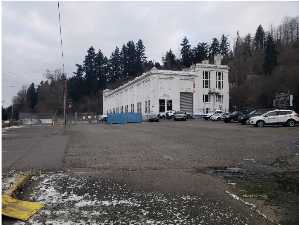
Photo 13 Typical view of a north-adjointing property to Parcel B (2111 E Valley Highway E), facing north from the southwest portion of Parcel B.
