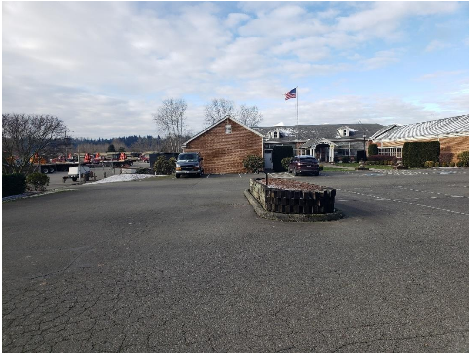
Photo 23 Typical view of the west-adjointing parent parcel (1808 E Valley Highway E), facing west from Parcel A.
