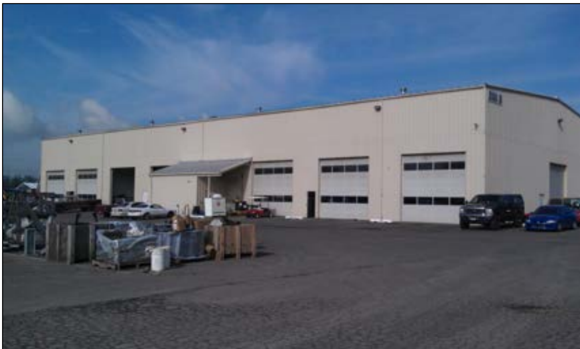
Photograph 6: Petersen Brothers truck maintenance building, Building B.
