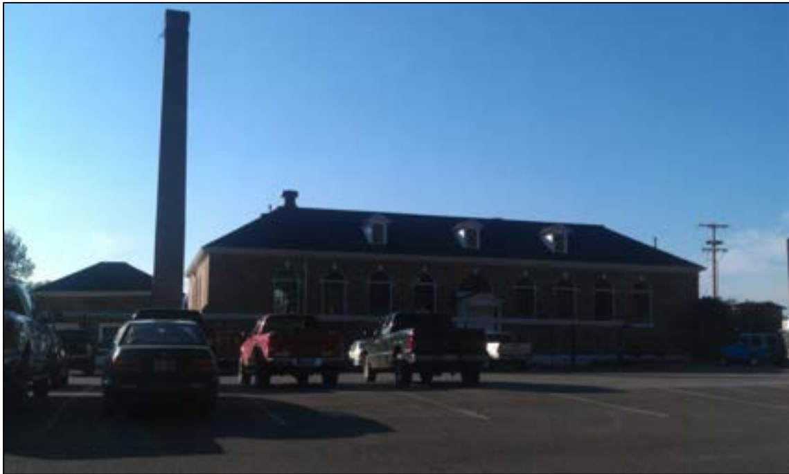
Photograph 13: Gymnasium on the northern Site parcel.
