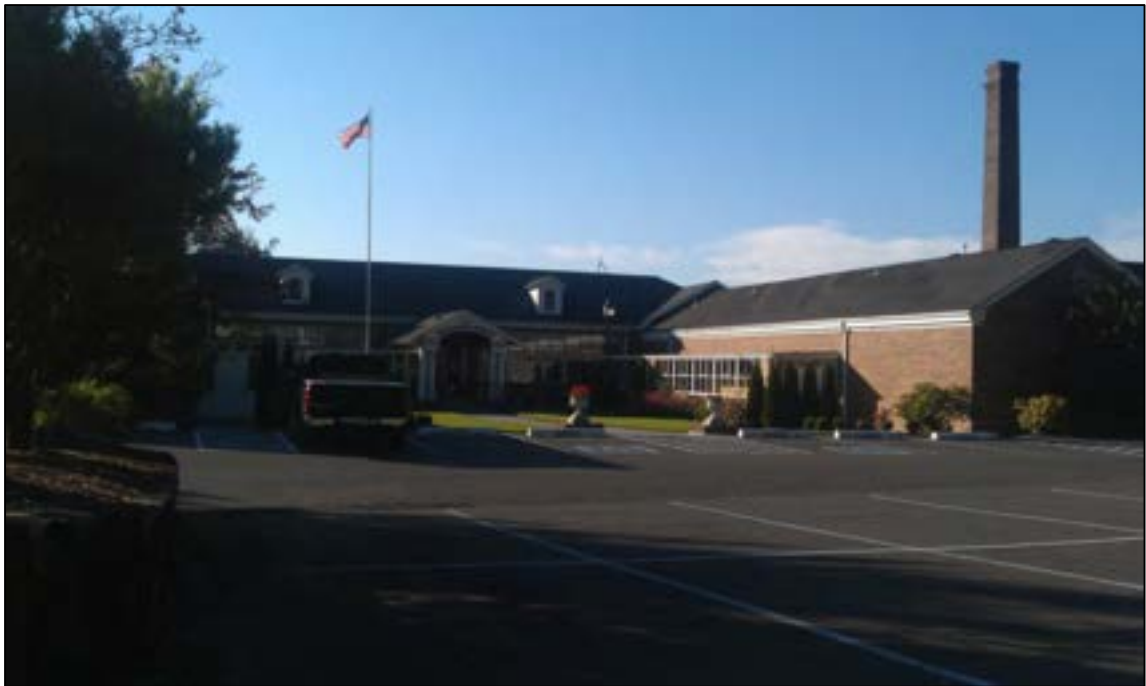
Photograph 12: Dieringer Business Park (former school) on the northern Site parcel.
