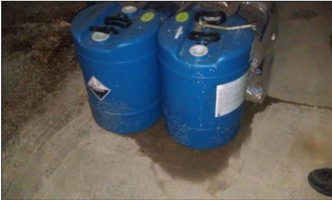
Photograph 43: Pool chemicals stored in gymnasium crawlspace.
