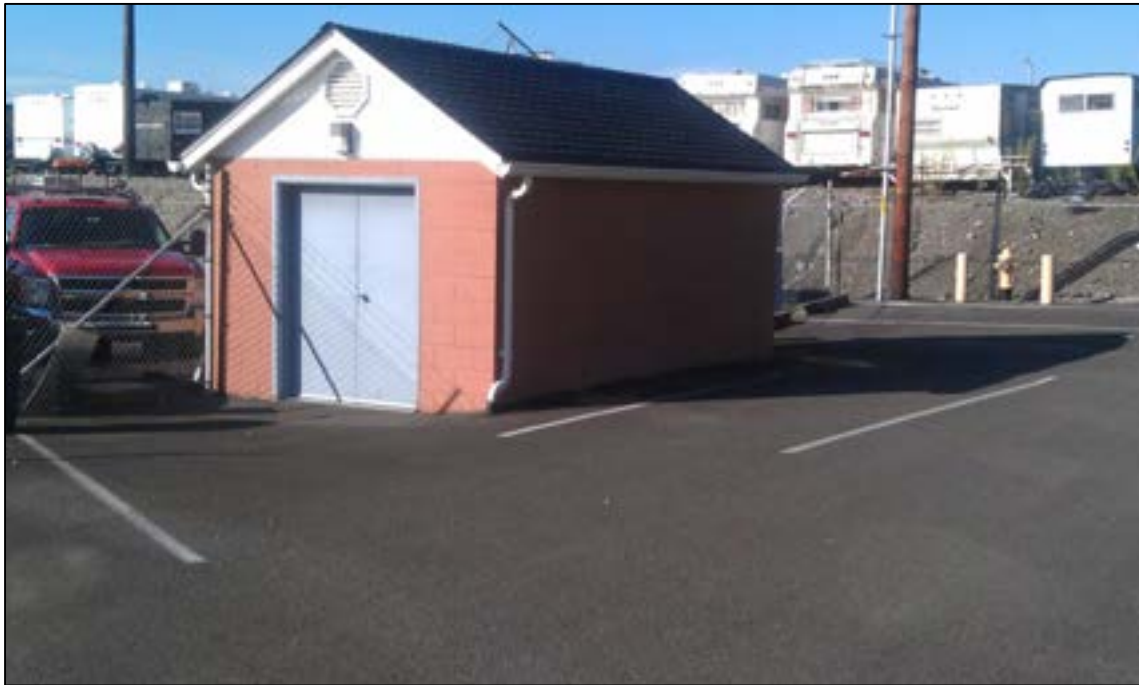
Photograph 15: City of Sumner well house.
