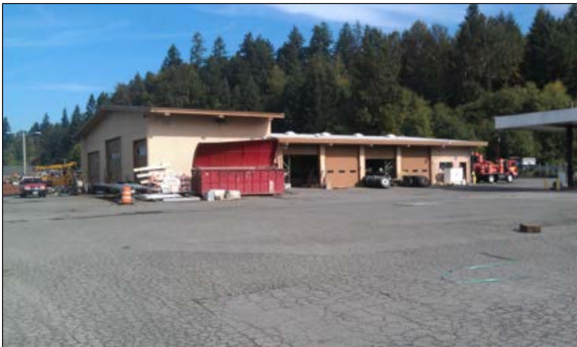
Photograph 8: Petersen Brothers storage warehouse (former truck maintenance building), Building A.
