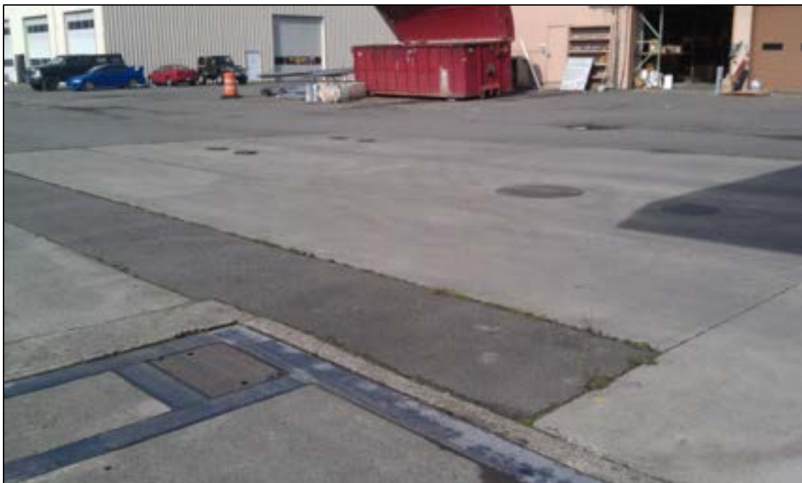
Photograph 10: Underground storage tank nest.
