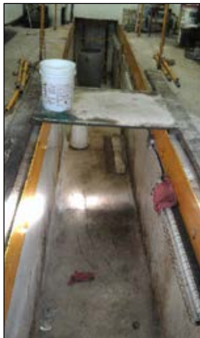
Photograph 28: Work pit observed in Building A service bay.
