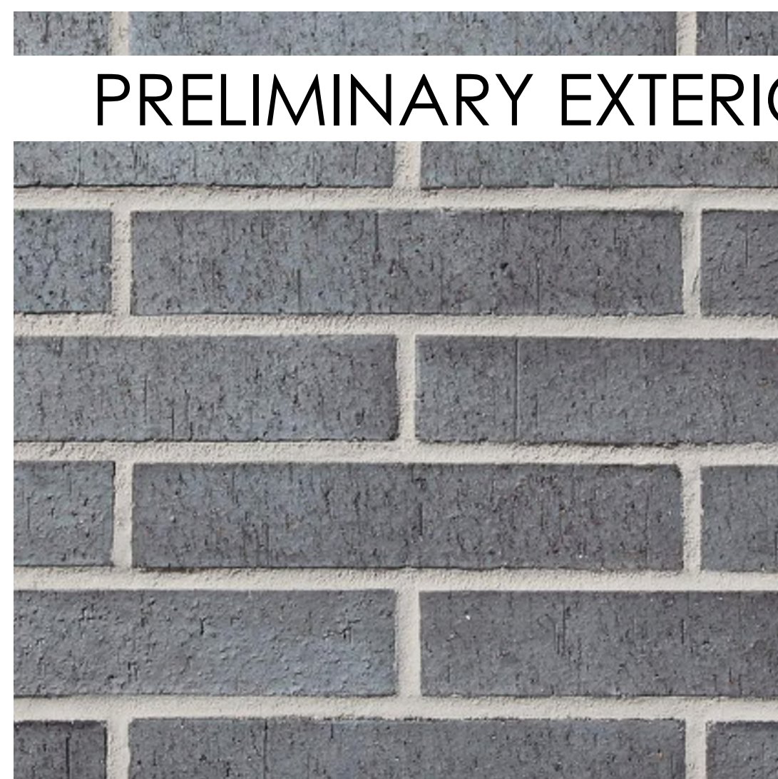
TYP BRICK - DARK GRAY CLINKER NORMAN THIN BRICK, RUNNING BOND (PACIFIC CLAY THIN BRICK IN DARK IRON SPOT or INTERSTATE THIN BRICK IN PLATINUM)
